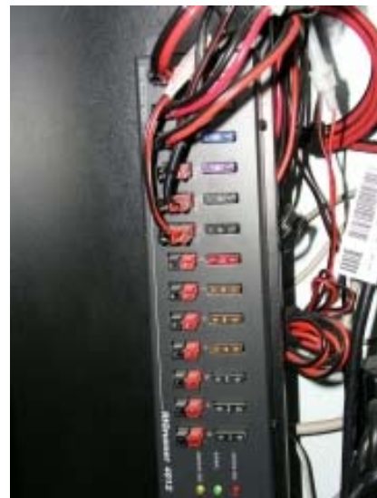
Making Connections to a Powerpole equipped DC Power Panel
