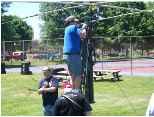
ASSEMBLING THE BEAMS
