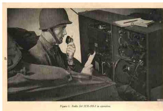
*Figure 1. Radio Set SCR-193-J in operation.*
